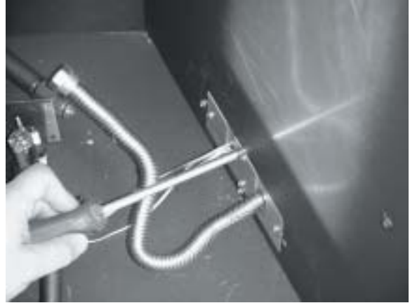
INSTALL SCREWS TO SECURE INLET BOX
