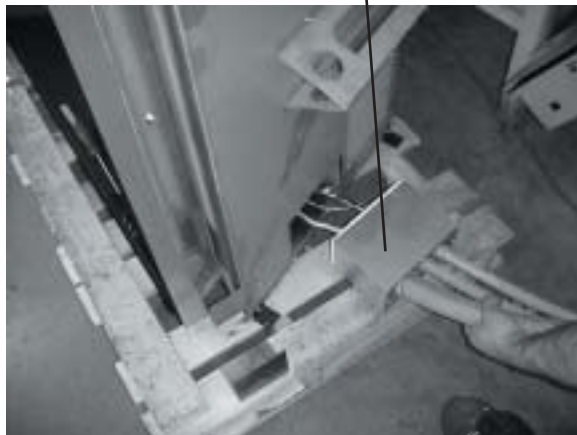
INSERT CONTROL ASSEMBLY
