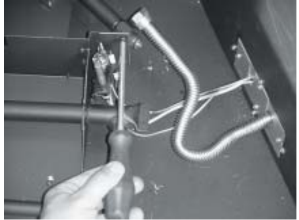
ATTACH PILOT BRACKET TO BURNER ASSEMBLY
