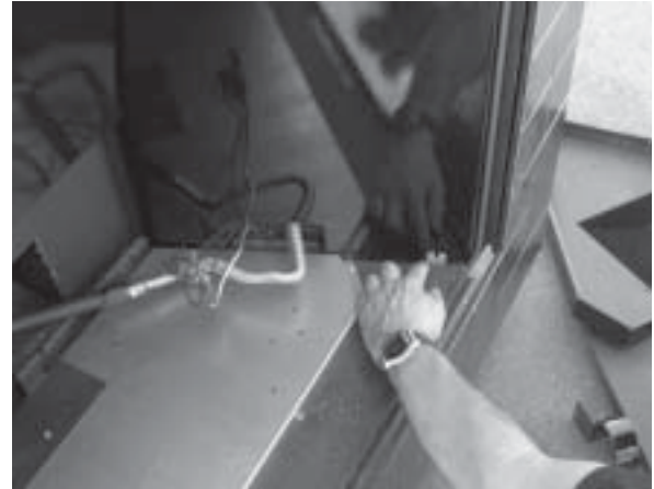
POSITIONING PANEL CLIPS
