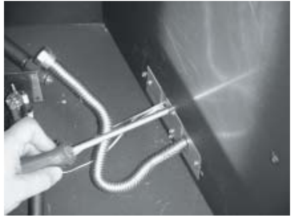
INSTALL SCREWS TO SECURE INLET BOX
