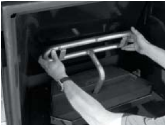
BURNER INSTALLATION
