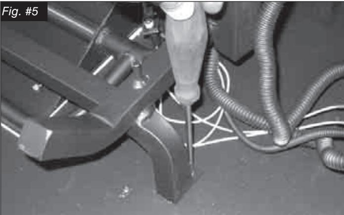
5. Position the grate and attach it to the floor with two screws located behind the front legs. (Fig. # 5)
