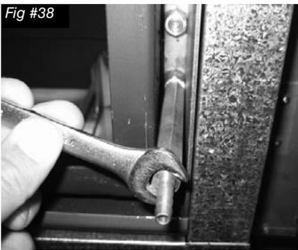
2. Thread the extension test fitting into the open port. (Fig. #38)
