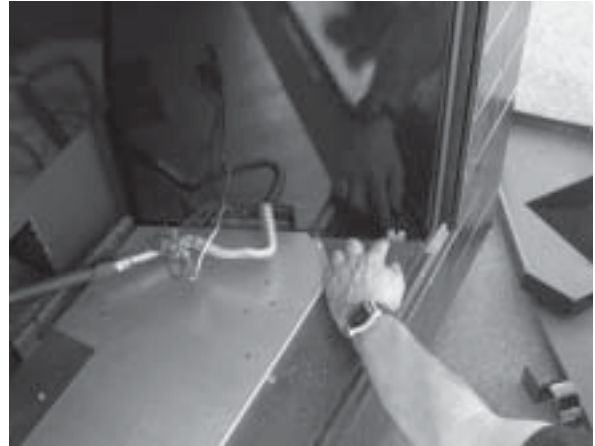
POSITIONING PANEL CLIPS
