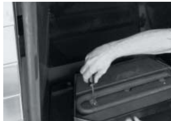
BURNER INSTALLATION
