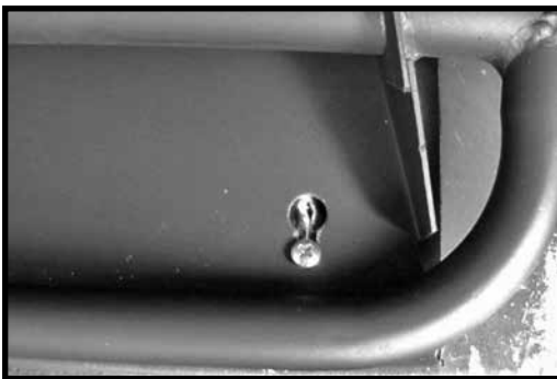
Figure 2: Attaching burner to floor of fireplace.
