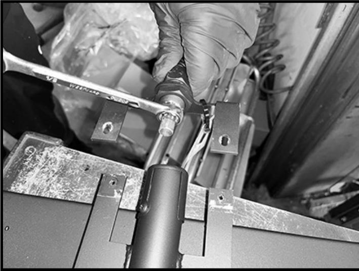
Figure 19: Removing orifice.
