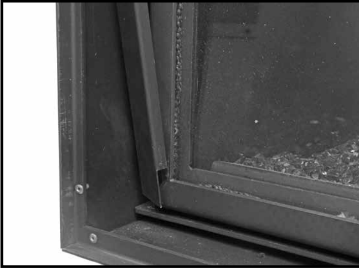
Figure 56: Installing the side trim.
