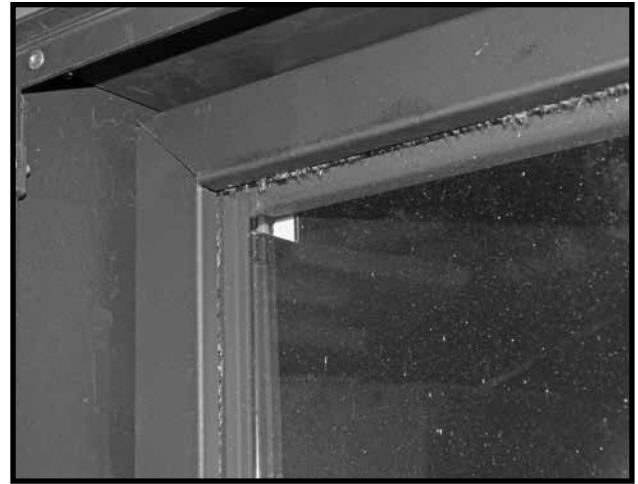
Figure 68: Top trim in place.
