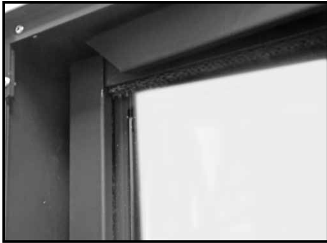
Figure 67: Installing top trim.
