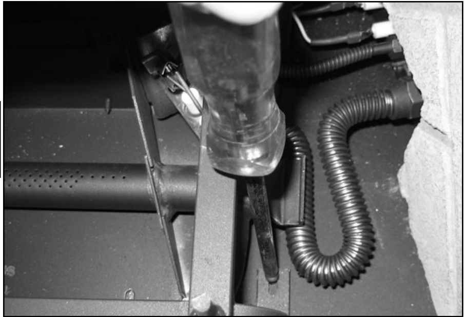
Figure 6: Attach log grate to floor.
