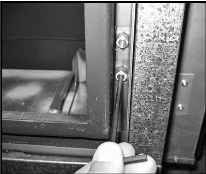
Figure 25: Removing manifold pressure plug.
