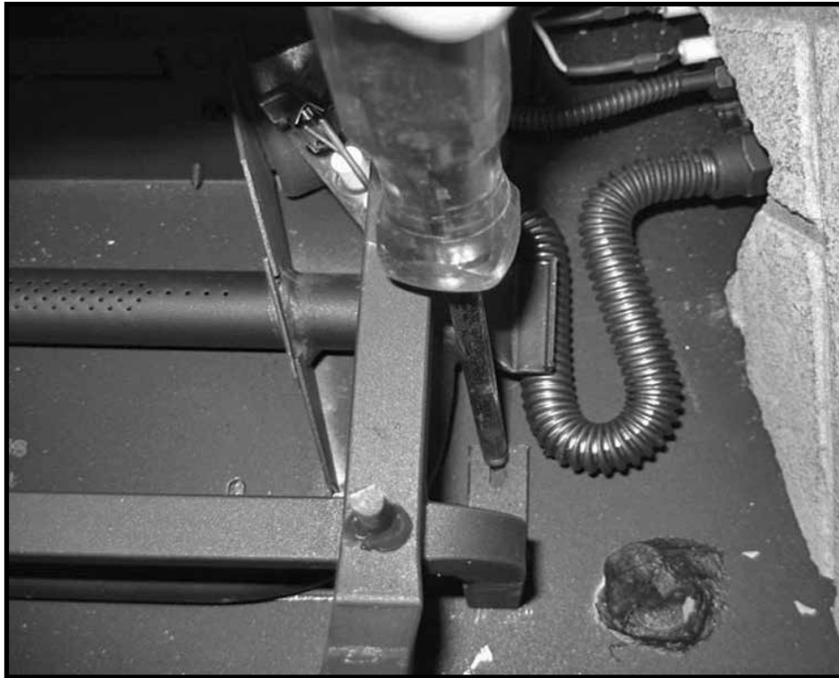
Figure 9: Securing log grate to the floor.
