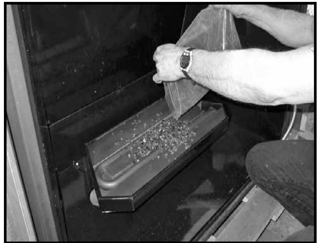
Figure 26: Applying glass media.
