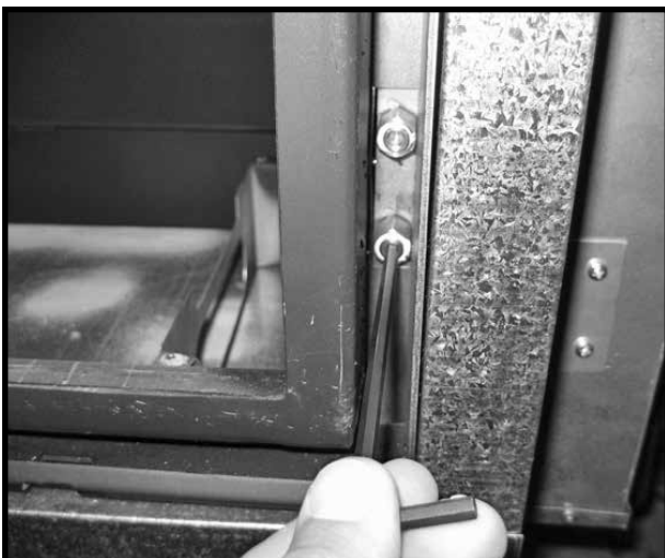
Figure 36: Removing manifold pressure plug.
