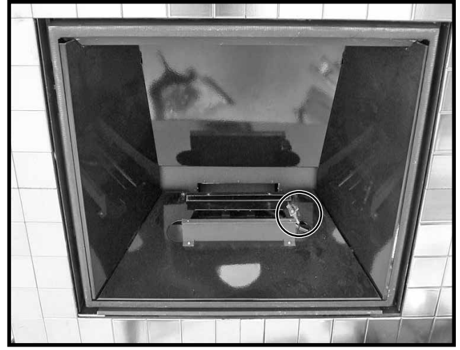
Figure 18: TC30 Pilot location.
