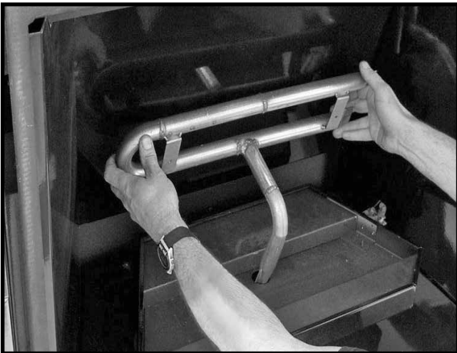
Figure 23: Burner installation.
