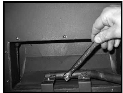
Figure 29: Removing natural gas orifice.
