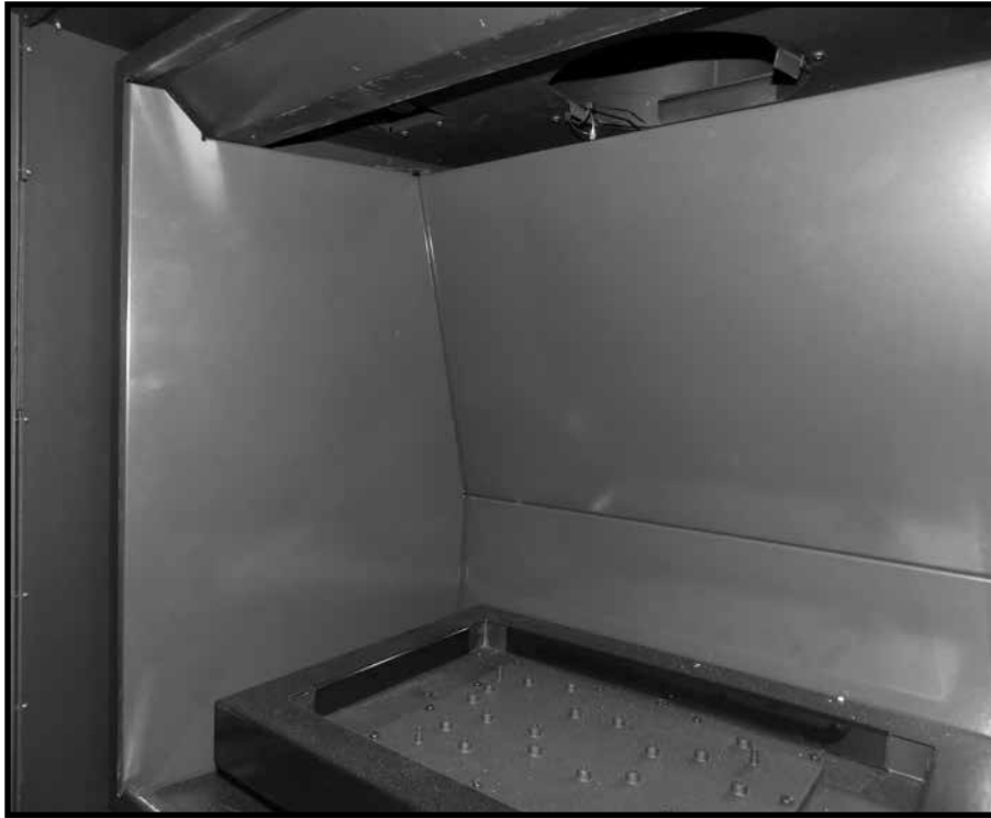
Figure 16: Left hand side panel installed.
