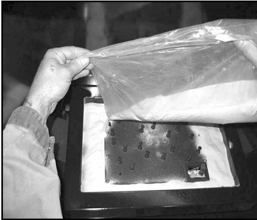
Figure 20: Applying sand to burner tray.
