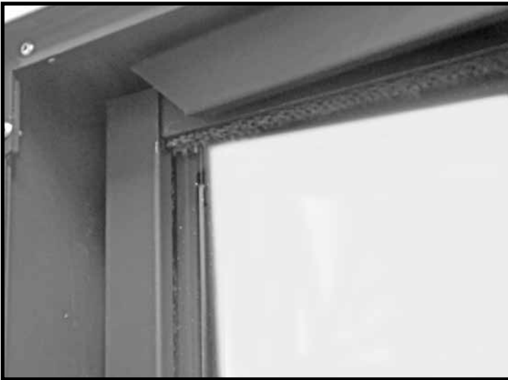
Figure 56: Installing top trim.
