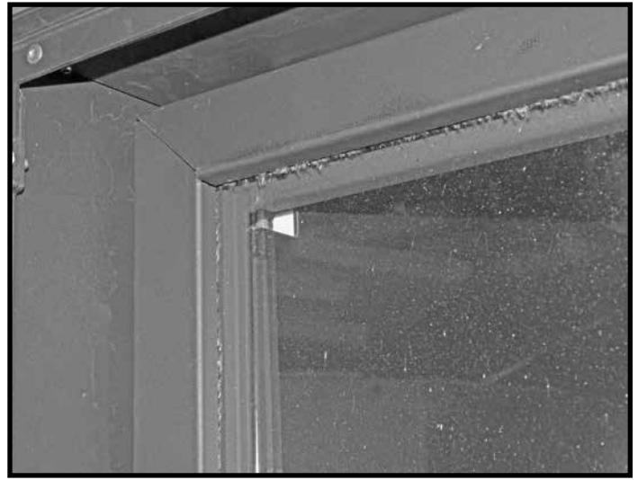
Figure 57: Top trim in place.
