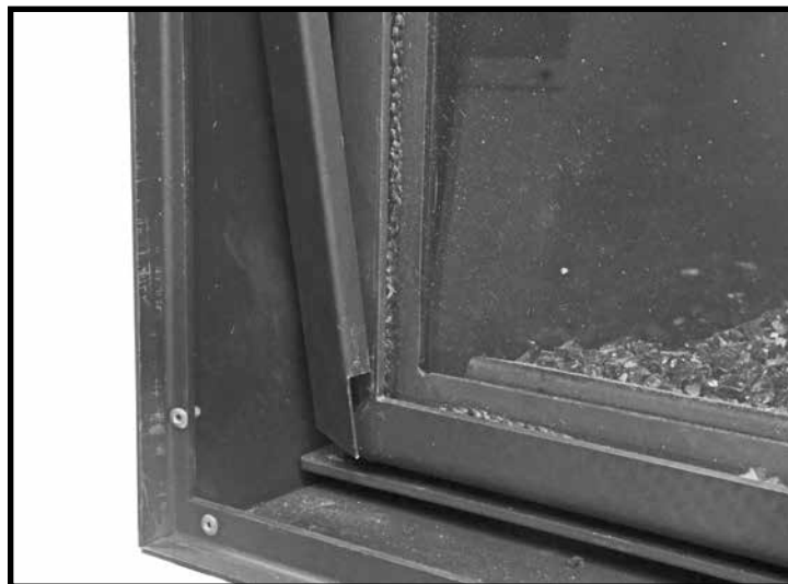
Figure 54: Installing the side trim.
