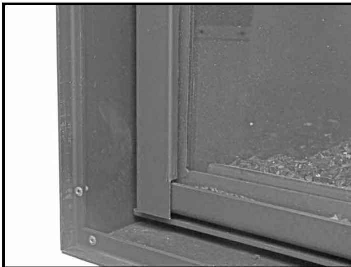
Figure 55: Side trim in place.
