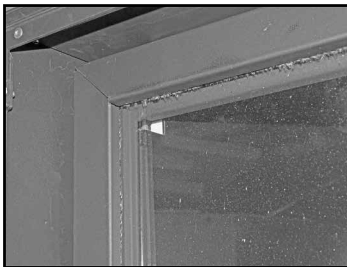
Figure 57: Top trim in place.
