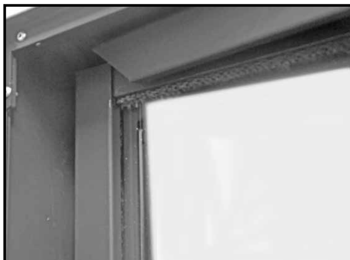
Figure 56: Installing top trim.
