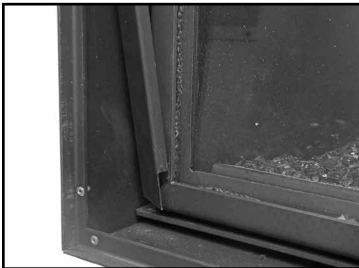
Figure 67: Installing the side trim.
