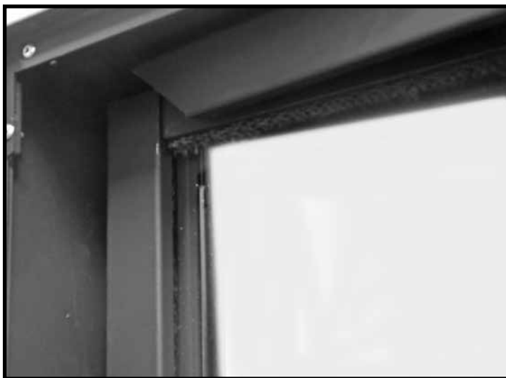
Figure 69: Installing top trim.
