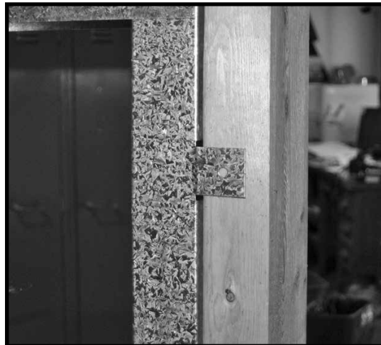
Figure 19: Attaching metal tab to frame
