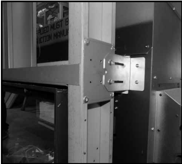
Figure 16: Framing bracket positioning.
