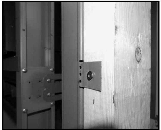
Figure 17: Attach tab to wood framing.
