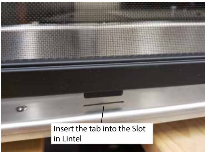
Figure 46: Screen Tab install.
