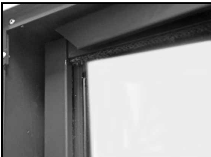
Figure 82: Installing top trim.
