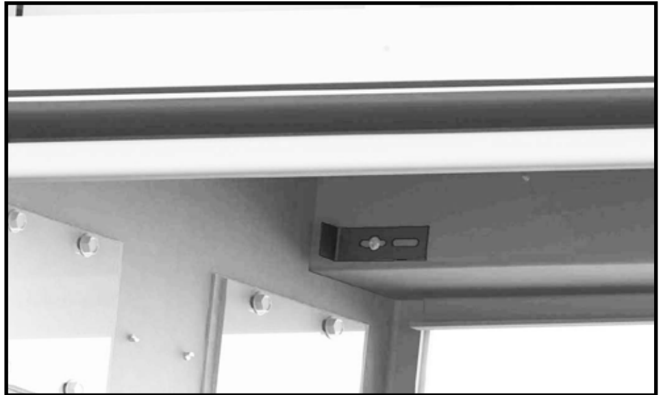
Figure 76: Panel retainer clip.
