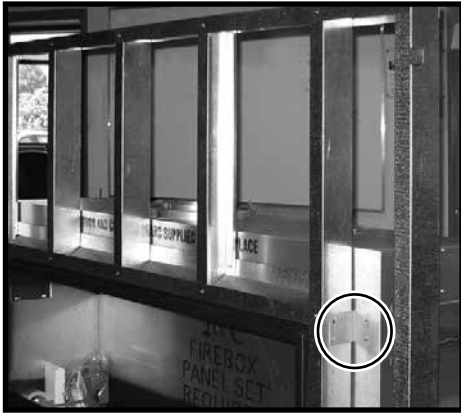
Figure 18: Framing Kit Brackets.
