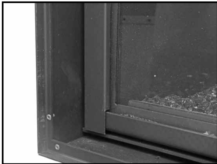
Figure 81: Side trim in place.
