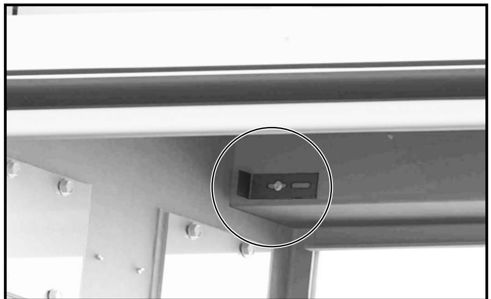
Figure 46: Panel retainer clip.
