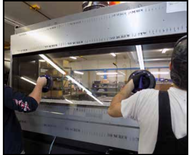
Figure 44: Installing inner glass sheet.
