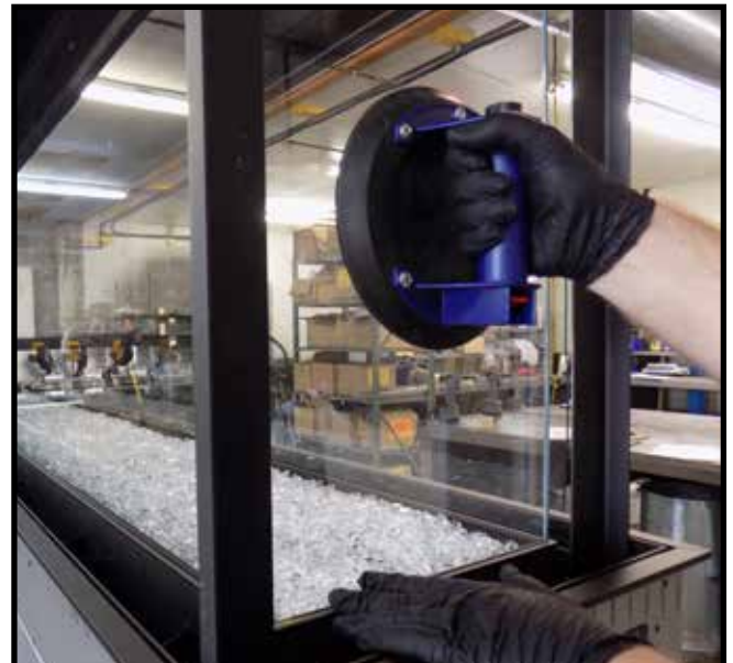
Figure 46: Installing inner end glass sheet.
