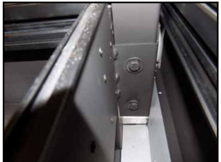
Figure 10: Lower support bolts to be removed.
