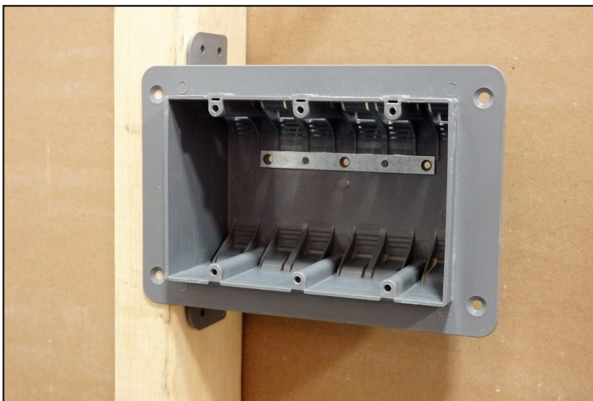
Figure 1: Plastic Electrical Box
