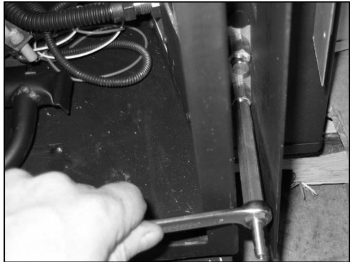
Figure 28: Adjusting manifold pressure.
