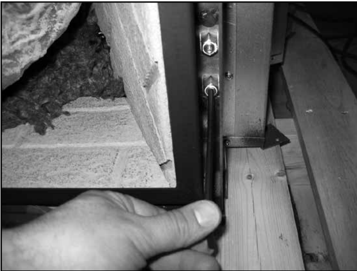
Figure 27: Removing manifold pressure plug.
