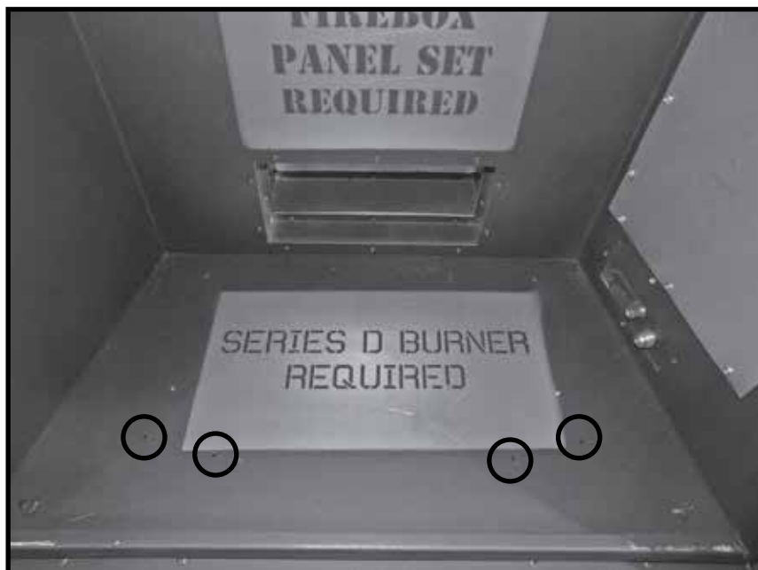
Figure 3: Removing floor shield.
