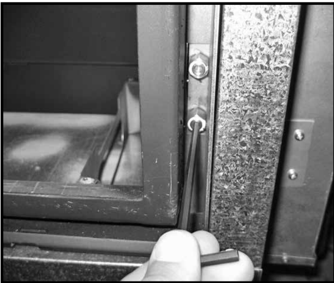
Figure 41: Removing manifold pressure plug.
