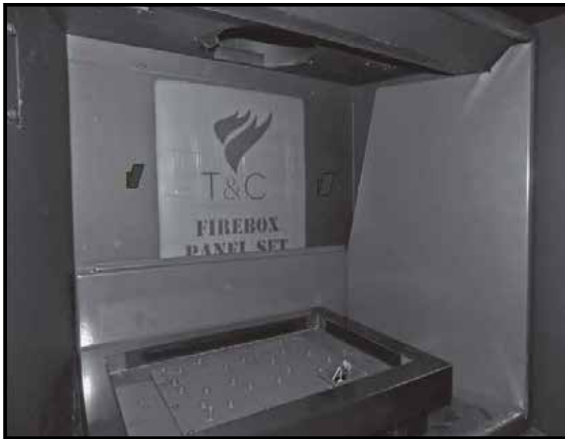
Figure 18: Right side panel partially installed.
