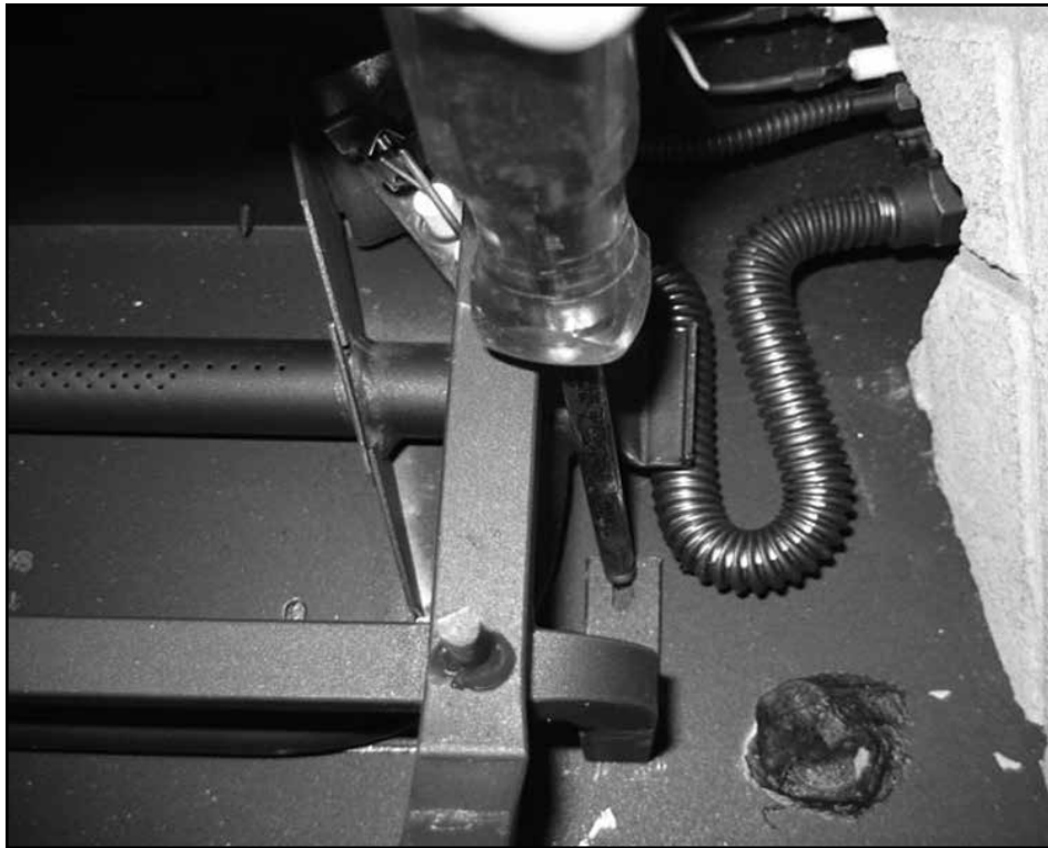
Figure 9: Securing log grate to the floor.
