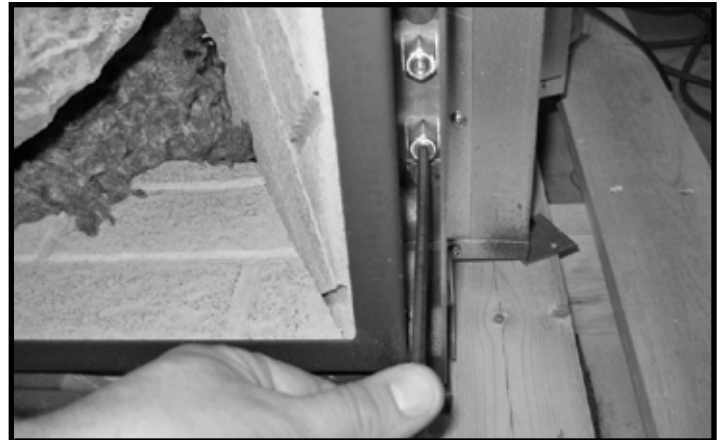
Figure 45: Removing test port plug.
