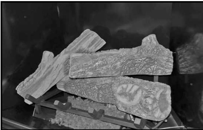
Figure 26: Third log placement.
