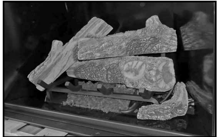
Figure 27: Fourth log placement.
