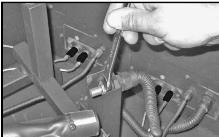
Figure 38: Replacing upper burner orifice.
