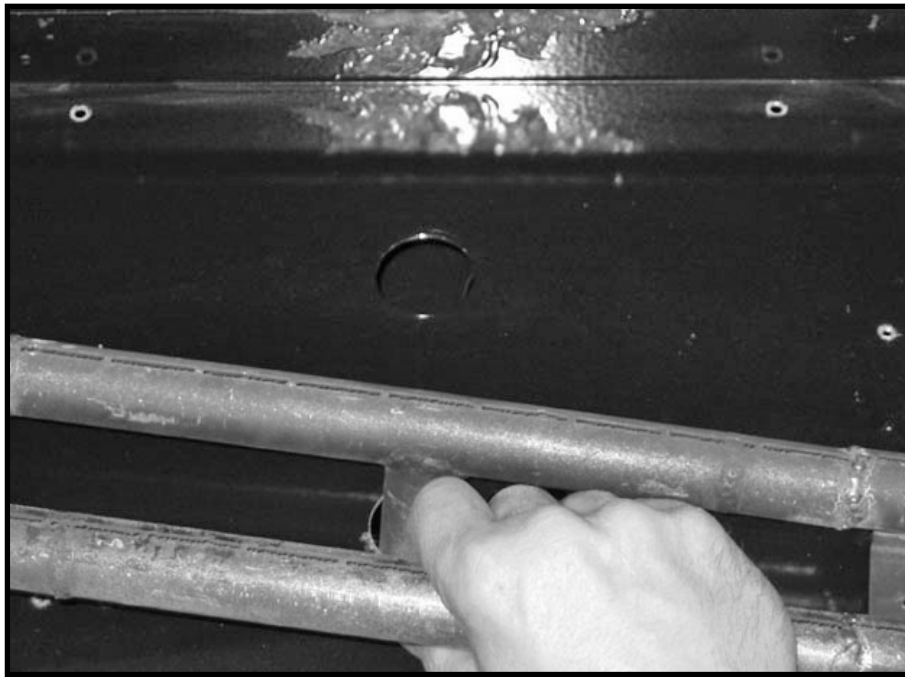
Figure 13: Installing front burner.
