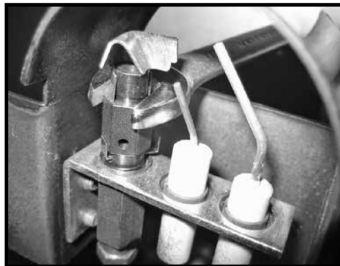
Figure 24: Loosen pilot head.
