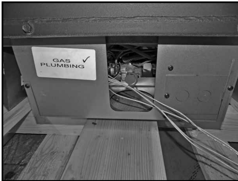
Figure 5: Lights wiring coming from grommet.
