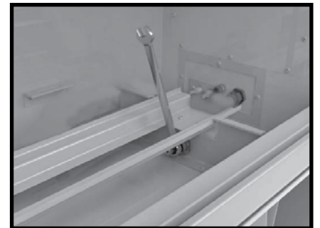
Figure 10: Installing the orifice.
