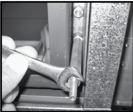
Figure 20: Gas pressure adjustment fitting.
