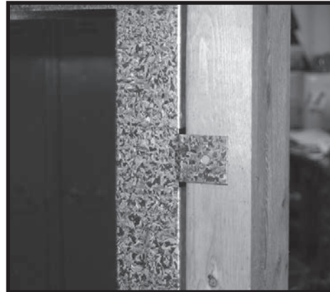
Figure 18: Attaching metal tab to frame.
