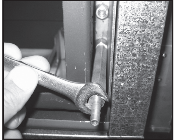
Figure 33: Installing pressure test extension.
