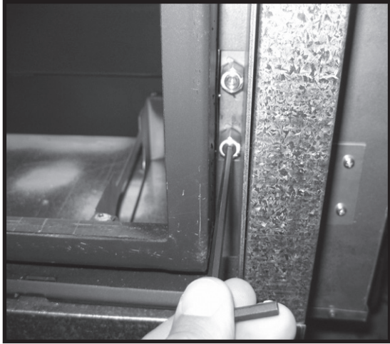
Figure 32: Removing pressure test plug.
