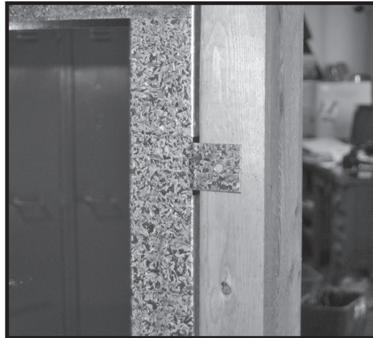
Figure 18: Attaching metal tab to frame.
