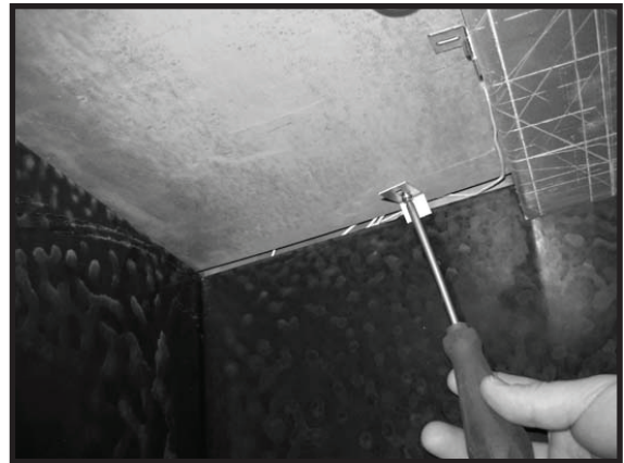
Figure 56: Side panel retainer.
