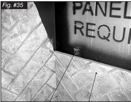
ADJUSTABLE "V" BRACKET REAR LOWER PANEL
