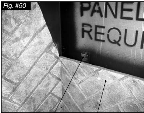
ADJUSTABLE "V" BRACKET REAR LOWER PANEL
