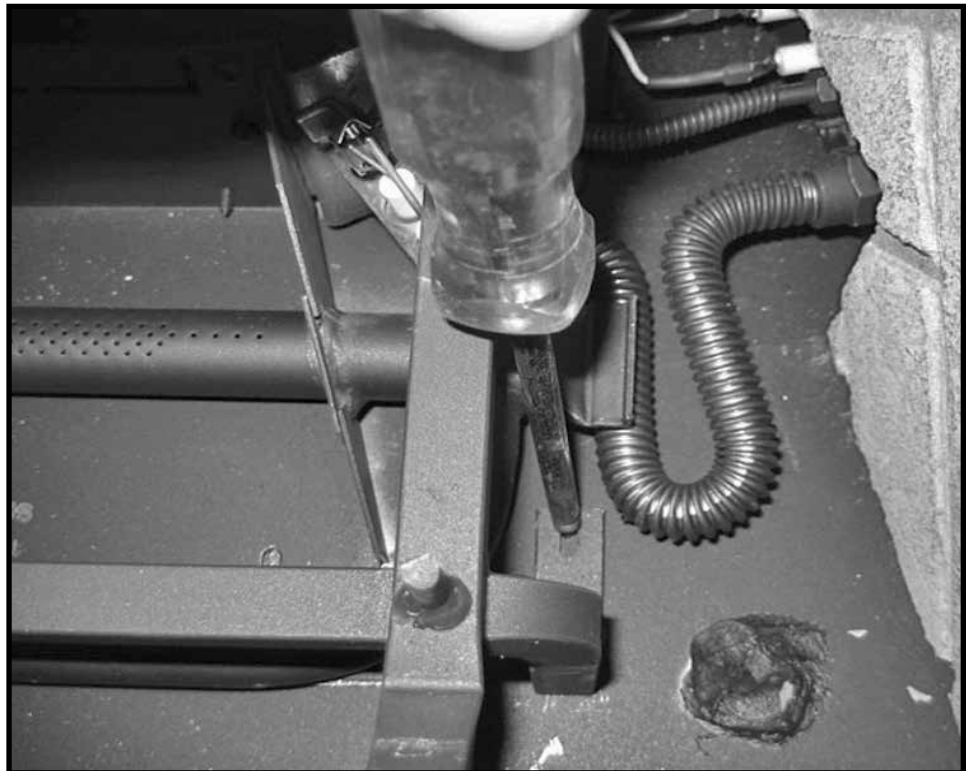
Figure 8: Securing the grate.
