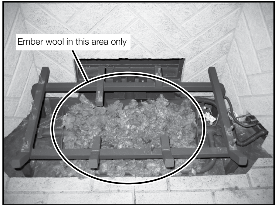
Figure 9: Placement of ember wool on the burner pan.
