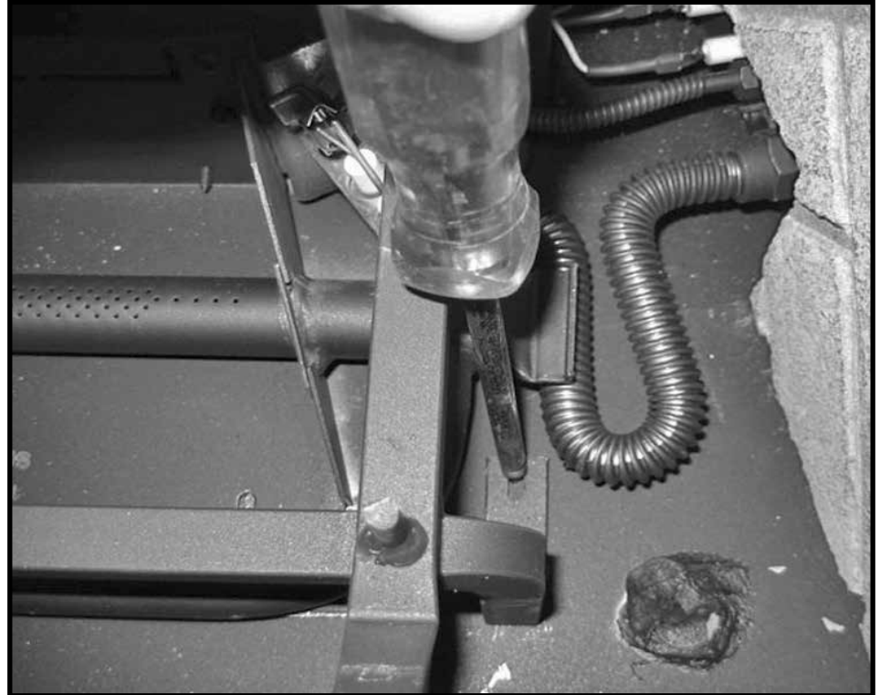
Figure 8: Securing the grate.
