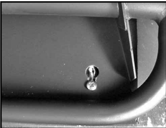
Figure 2: Attaching burner to floor of fireplace.
