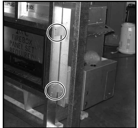
Figure 18: Framing bracket fastening points.
