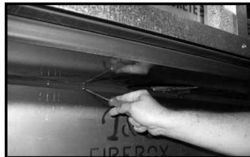
Figure 37: Securing top porcelain panel.
