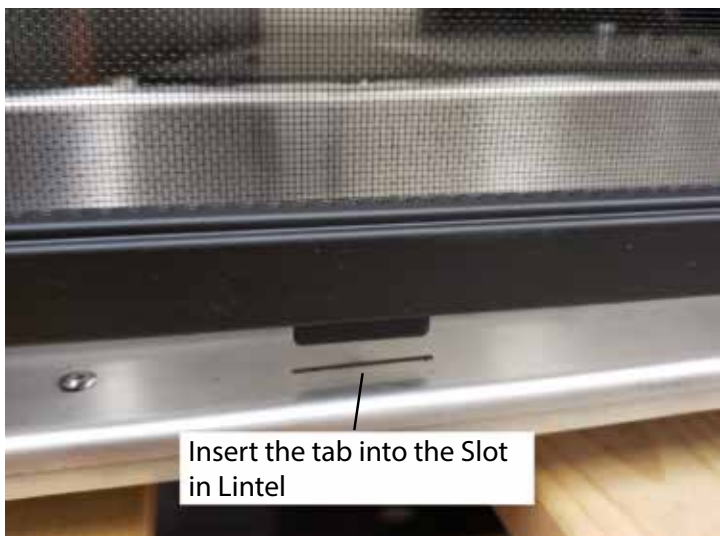
Figure 21: Screen Tab install.
