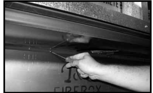
Figure 39: Securing top porcelain panel.
