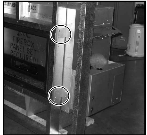
Figure 18: Framing bracket fastening points.
