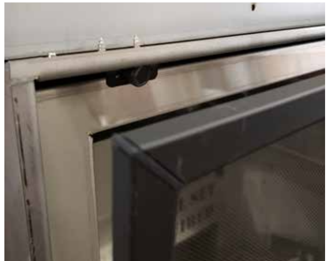
Figure 22: Screen Magnets.
