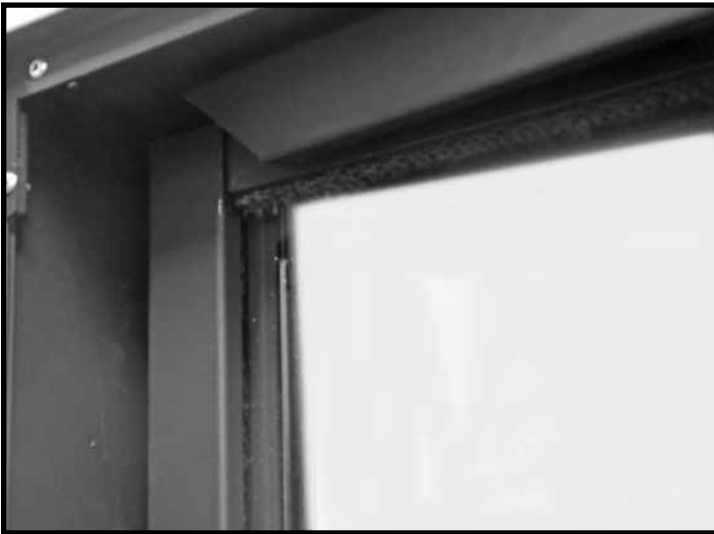
Figure 58: Installing top trim.
