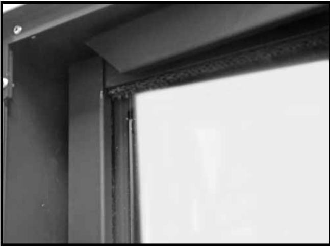
Figure 67: Installing top trim.
