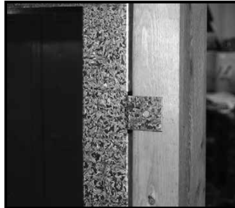
Figure 17: Attaching metal tab to frame.
