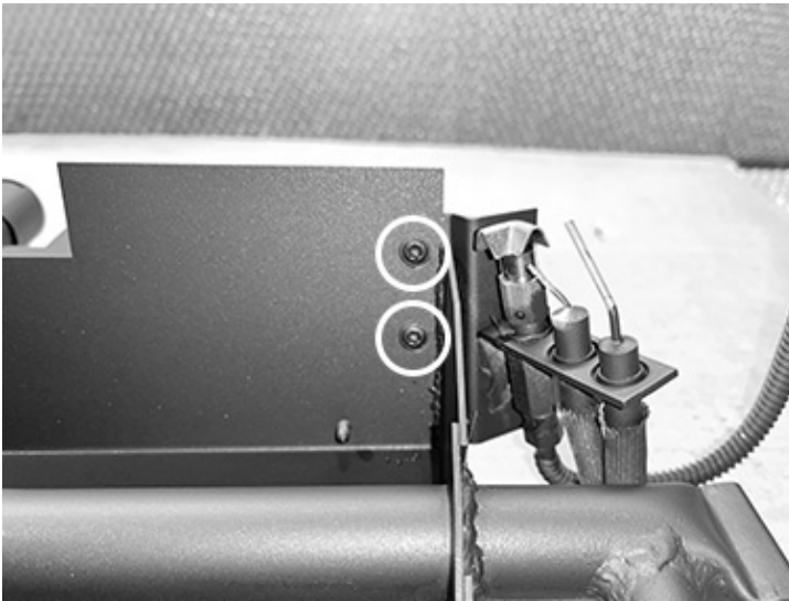
Figure 41: Remove burner pilot.
