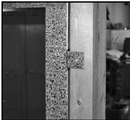
Figure 19: Attaching metal tab to frame
