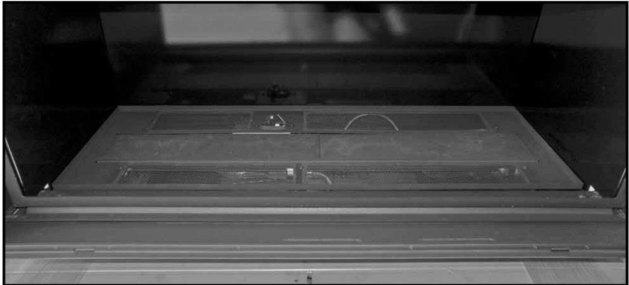
Figure 60: Burner tray installed and secured.
