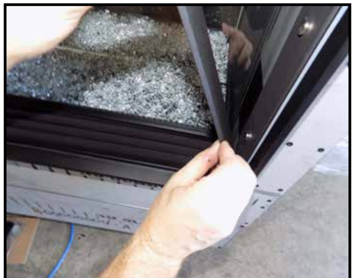
Figure 48: Installing right side securing plate.
