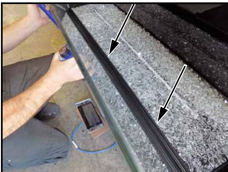
Figure 43: Lowering bottom edge of inner plate into gap.
