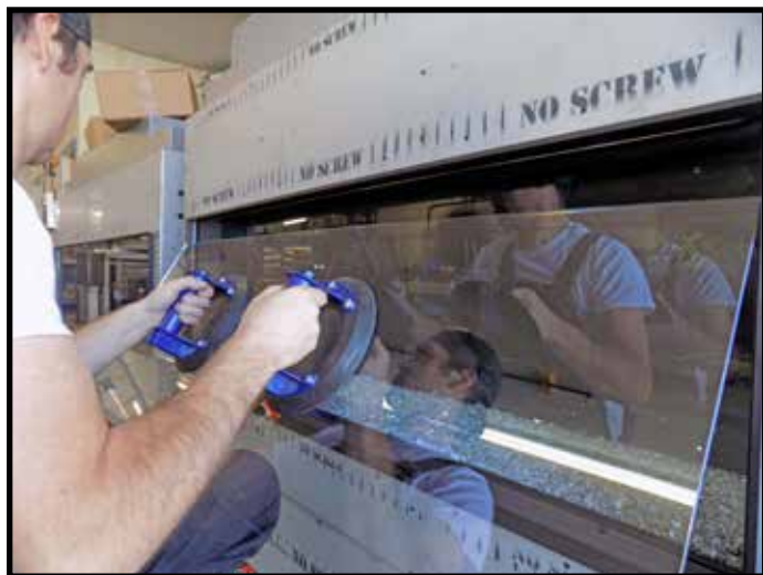
Figure 50: Insert top end of outer glass sheet in first.
