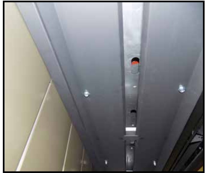
Figure 31: Adjustment accessible through the baffle cover.
