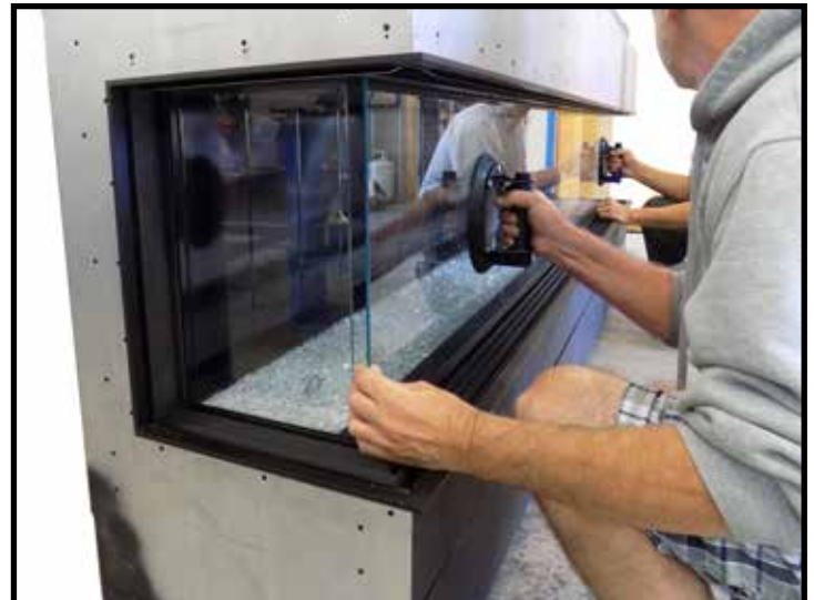
Figure 45: Installing the inside front glass plate.
