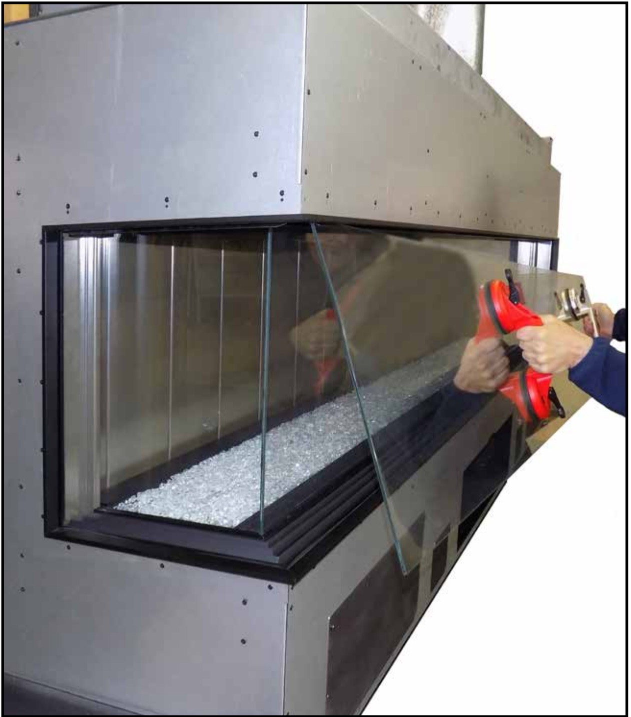
Figure 54: Inserting top edge of outside front plate.
