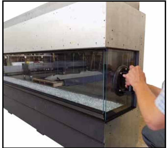
Figure 53: Installing outside right hand side plate.
