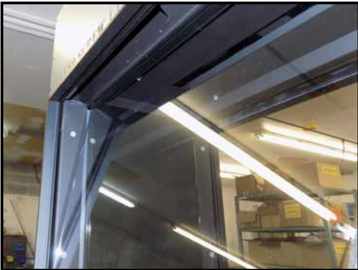
Figure 37: Top edge of sheet goes in first.
