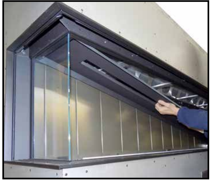
Figure 26: Installing baffle cover.
