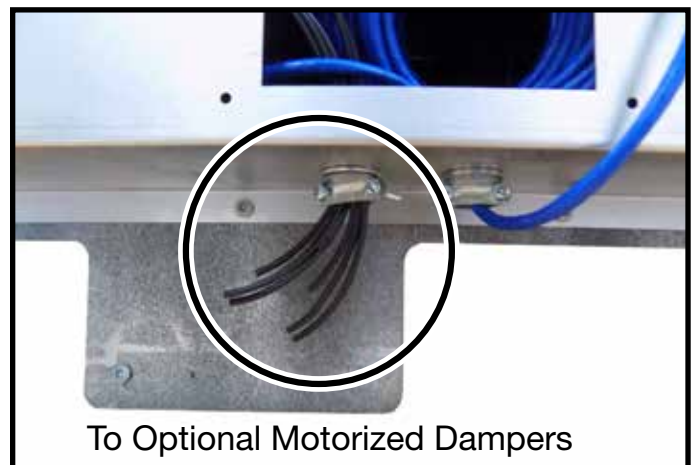
Figure 48: Motorized damper electrical connections.
