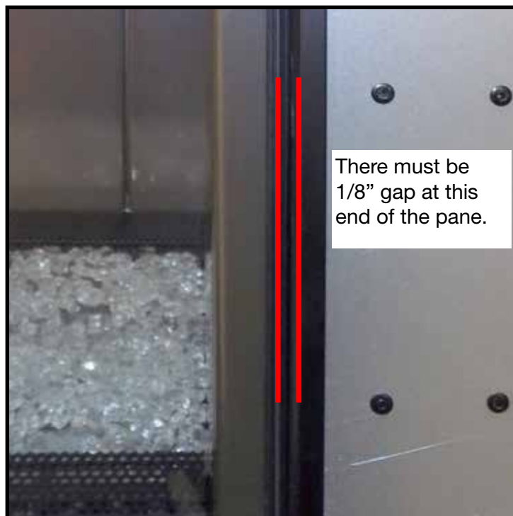
Figure 45: Gap on right side.
