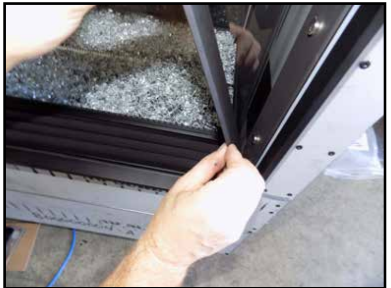
Figure 42: Installing right side securing panel.
