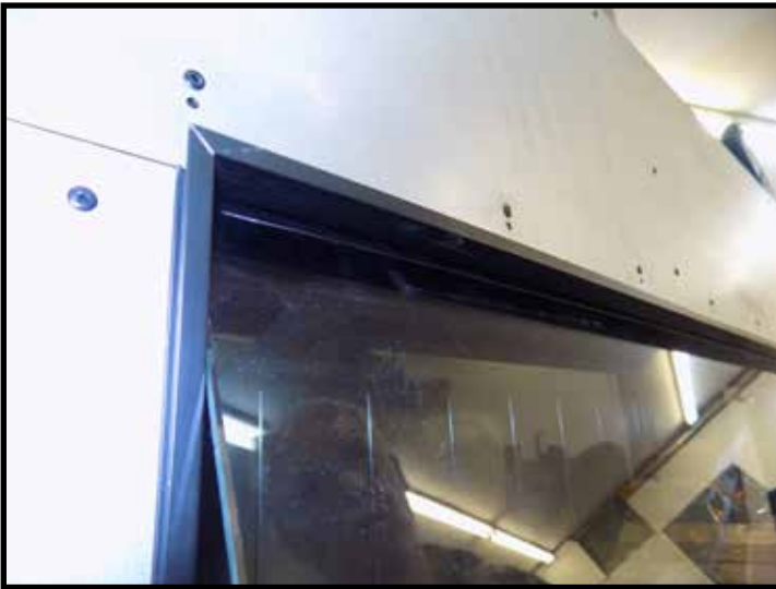
Figure 43: Inserting outside glass sheet.
