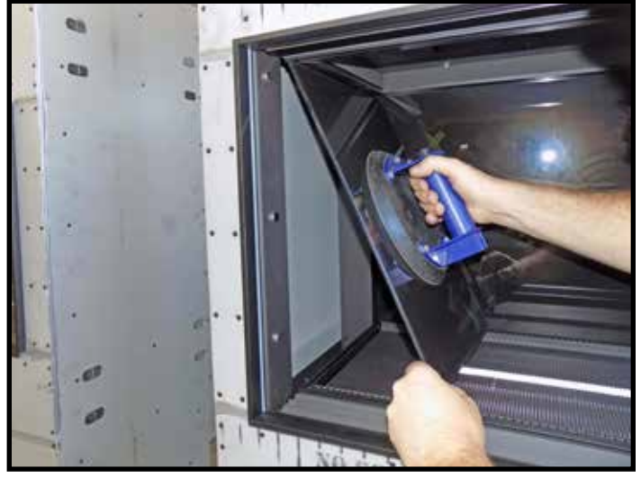
Figure 30: Insert top of side black glass first.
