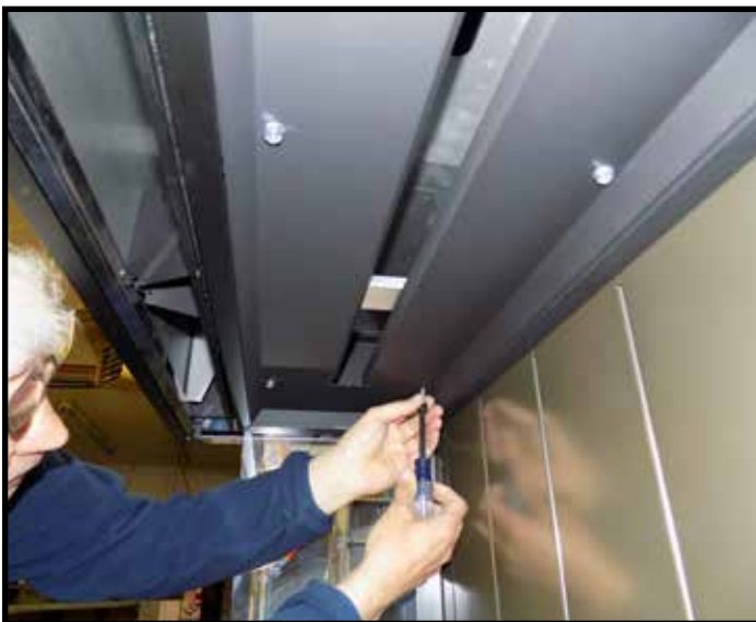
Figure 27: Securing the baffle cover.
