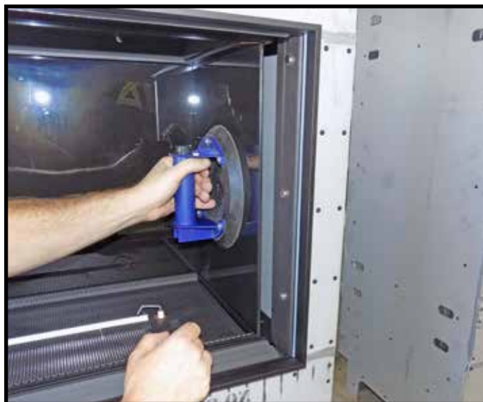
Figure 36: Insert bottom end of side black glass plate.
