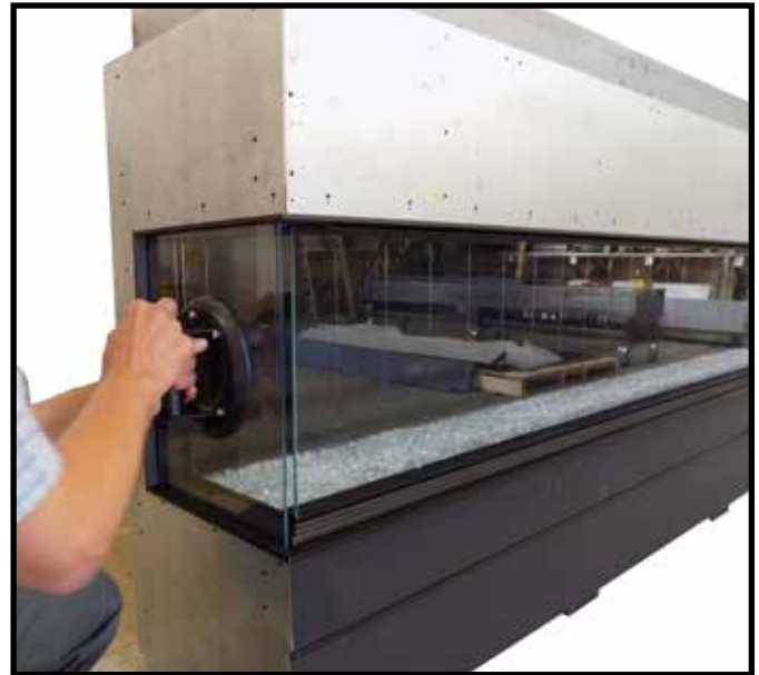
Figure 48: Lowering outside right hand side plate.
