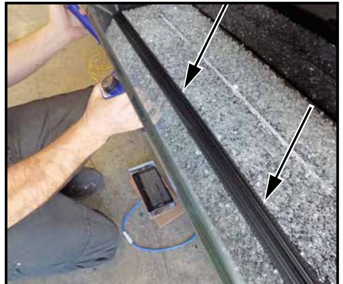
Figure 40: Lowering bottom edge of inner front plate into gap.
