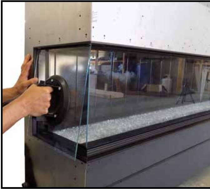
Figure 47: Installing outside right hand side plate.
