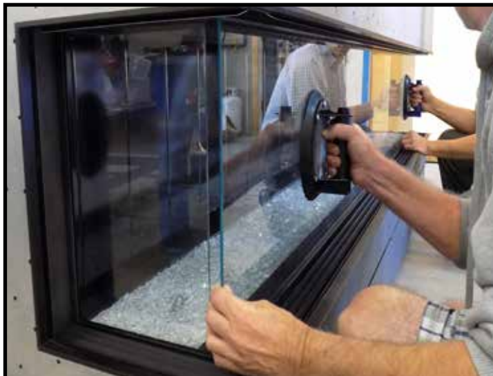
Figure 49: Installing the inside front glass plate.
