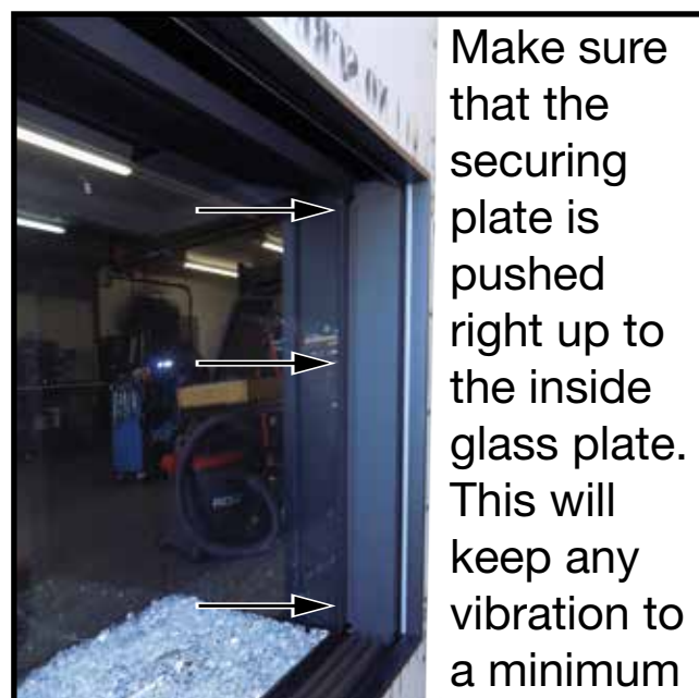
Figure 46: Position securing plate up against the inside glass plate.
