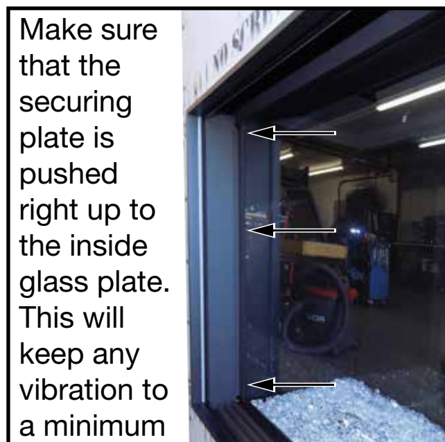
Figure 48: Position securing plate up against the inside glass plate.
