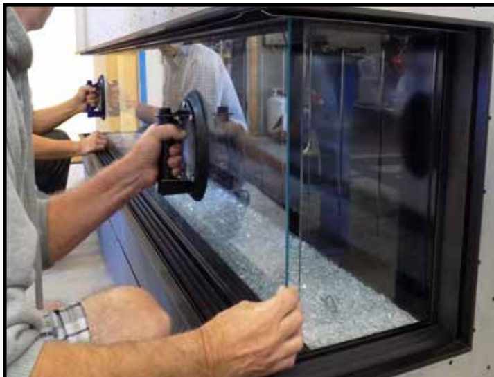
Figure 51: Installing the inside front glass plate.
