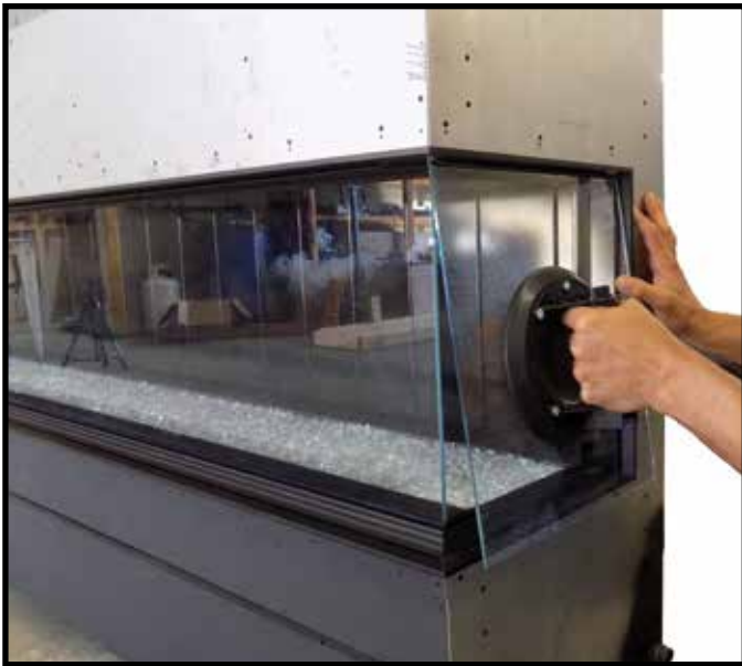
Figure 49: Installing outside right hand side plate.
